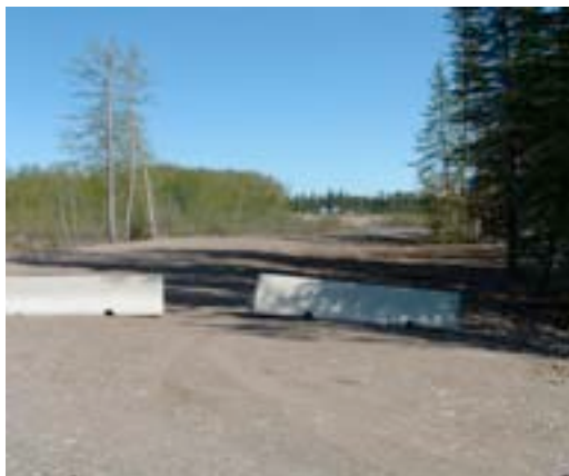
2007 Telkwa Phase III Dike
